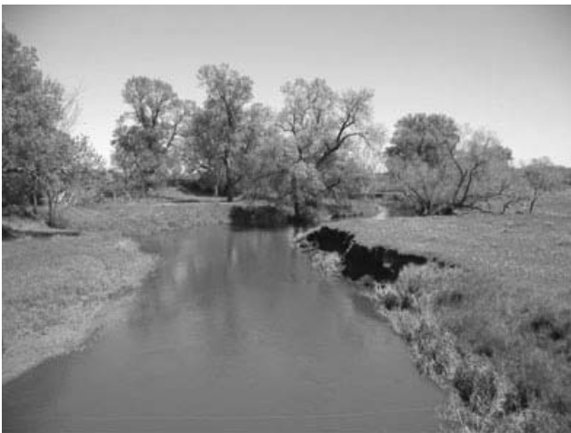
Figure 5. The photo shows slight entrenchment of an Elm Creek reach with a bank height ratio of about 1.3. The current active floodplain on the left of the photo lies 1–2 m below the terrace on the right. Following entrenchment, the channel has increased in width (as described in stage IV of the channel evolution model). Although entrenchment is slight, it is important because it reduced the frequency of overbank flooding. This figure is available in colour online at wileyonlinelibrary.com/journal/trra .
